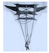
levers to control the "wings", thereby allowing the "pilot" to control the descent and land safely should the wire connecting the kite to the ground suddenly break.
